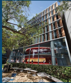
> Ainsworth Mechanical and Manufacturing Engineering and Precinct
